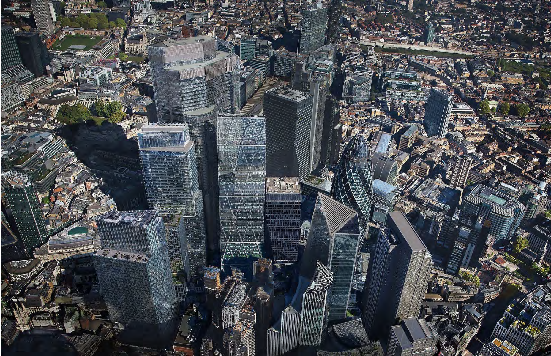
Aerial View of Site
